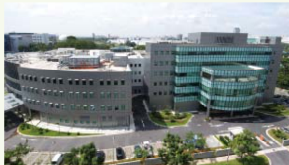
Exterior View of WaterHub
