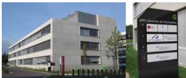
The exterior of the Nitto Denko Europe Technical Centre Sàrl (NET)
