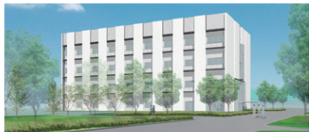
Kameyama Plant Technical Center
