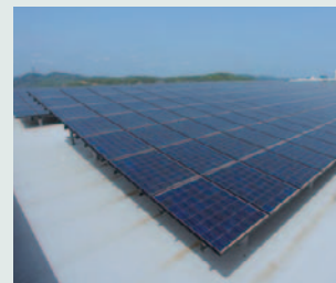
Solar generation system
