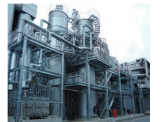
Solvent recovery equipment at the Toyohashi Plant
