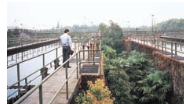
Industrial park wastewater treatment facilities in Shanghai
