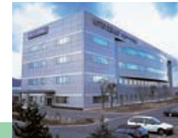
■ Adhesive Tape Research and Technology Center in Toyohashi plant
