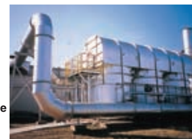
Catalyst deodorizing furnace at Nitto Denko (Shanghai Songjiang) Co., Ltd. (China)
