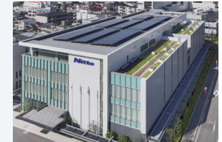
Solar power generation system on the roof
