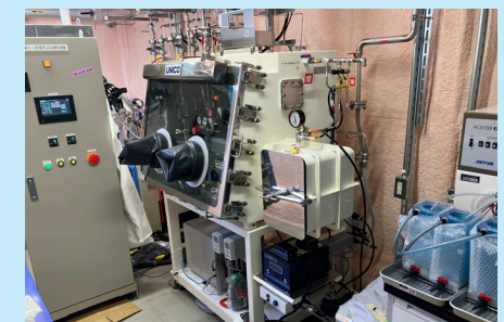
Formic acid production equipment
