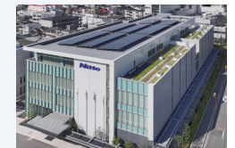
Solar power generation system on the roof
