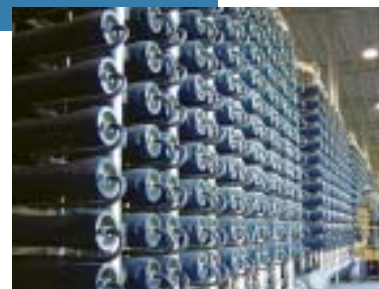
Seawater desalination plant
