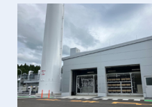
Hydrogen Utilization Facility
