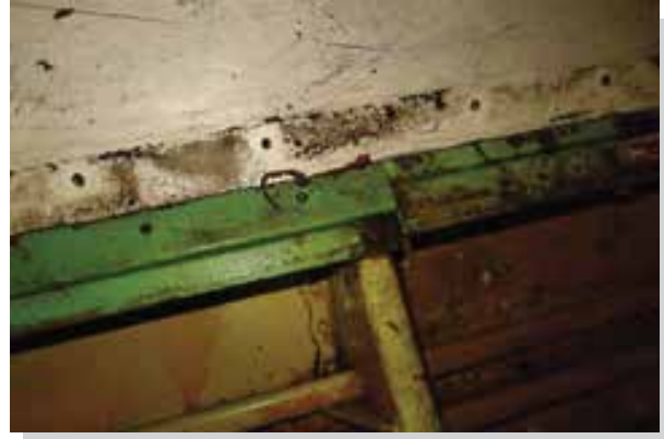
Aeroseal® SC-140 removed cleanly from floor structure
